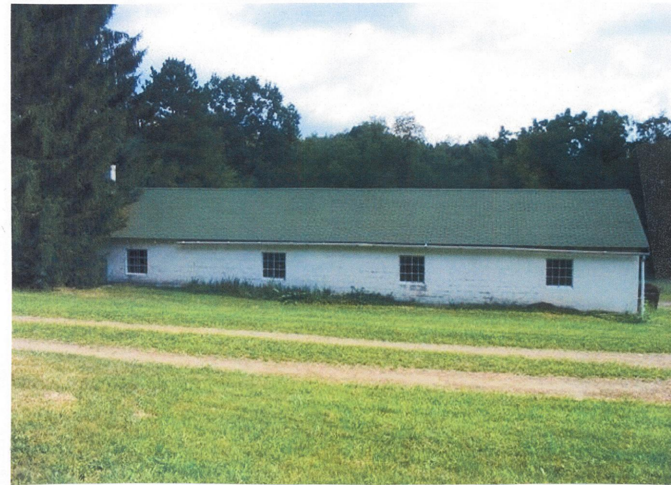
PICTURE OF BUILDING (SOUTH SIDE)
