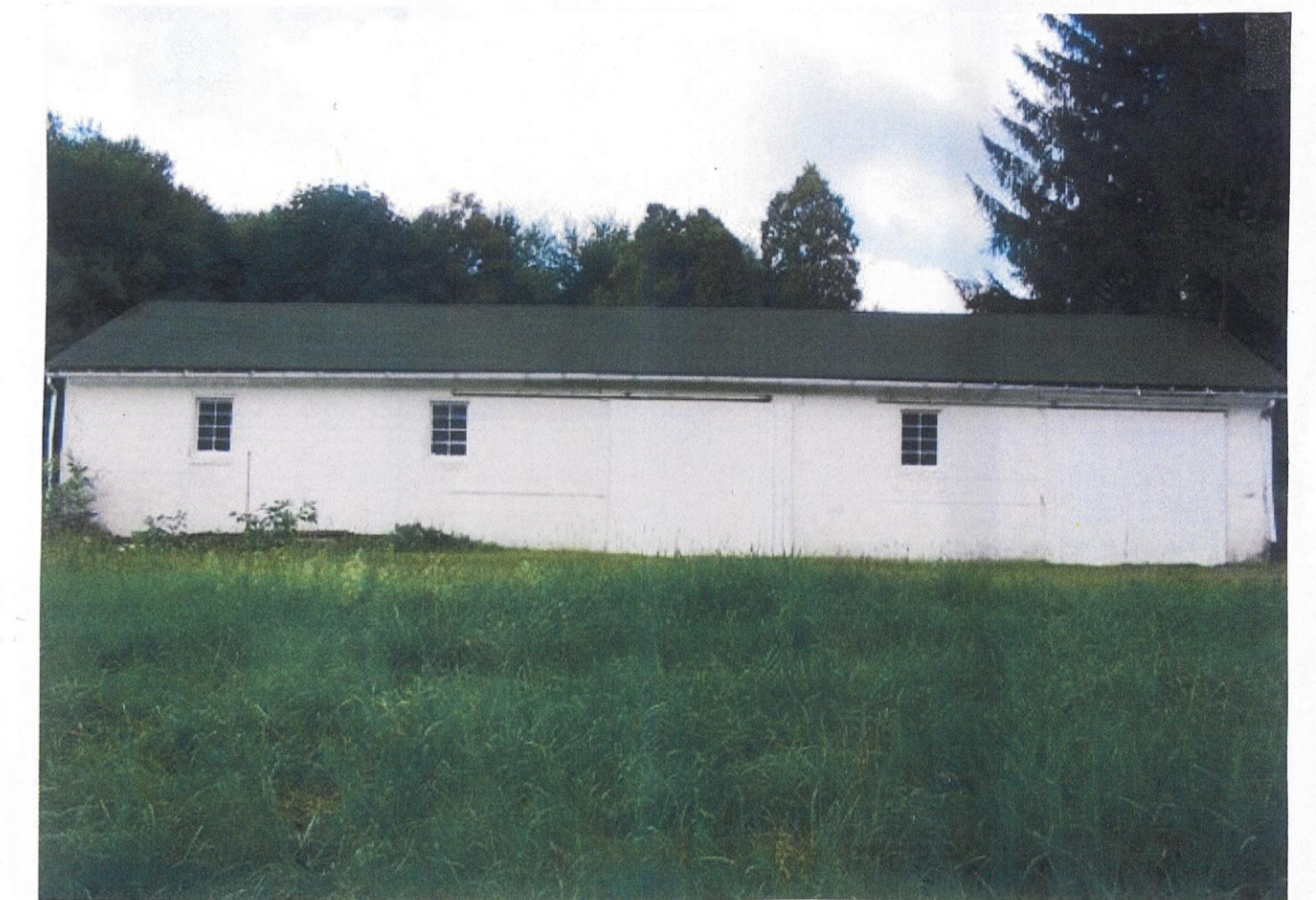
PICTURE OF BUILDING (NORTH SIDE)
