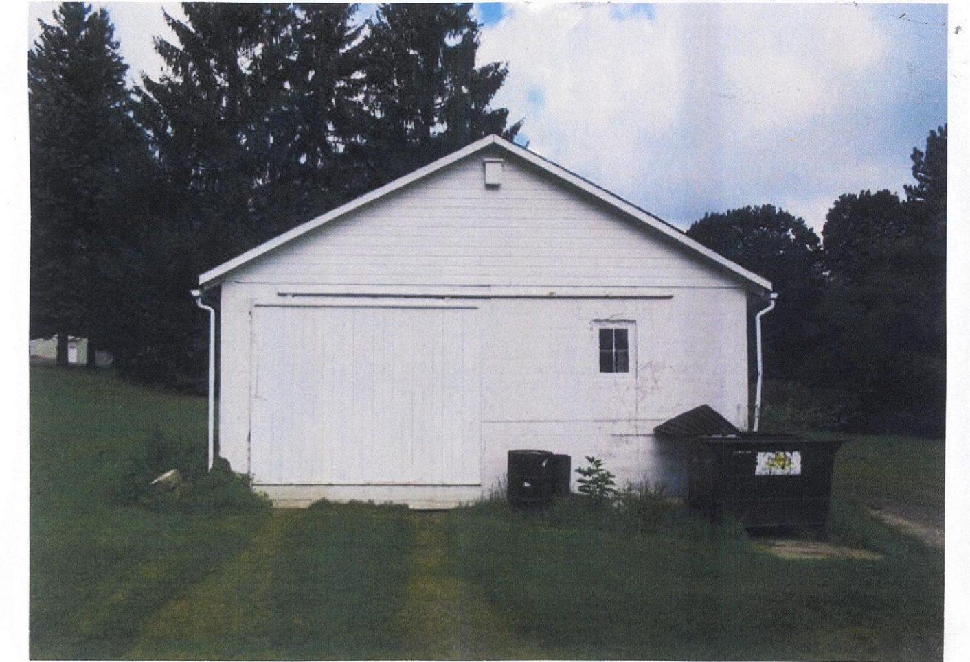
PICTURE OF BUILDING (EAST SIDE)
